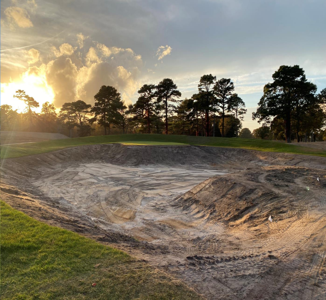
Hauling and shaping of new greenside bunker #16
